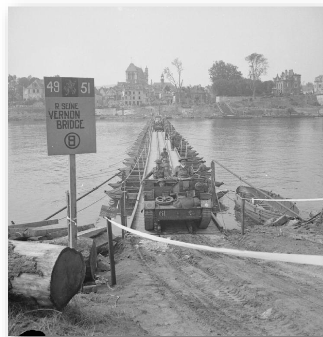
4th Dorsets cross 'David', the Class 9 FBE bridge across the Seine at Vernon, 27 August 1944. The numbers 49 and 51 either side of the Wessex Wyvern divisional badge are the identification serials of 204 and 553 Field Companies RE
