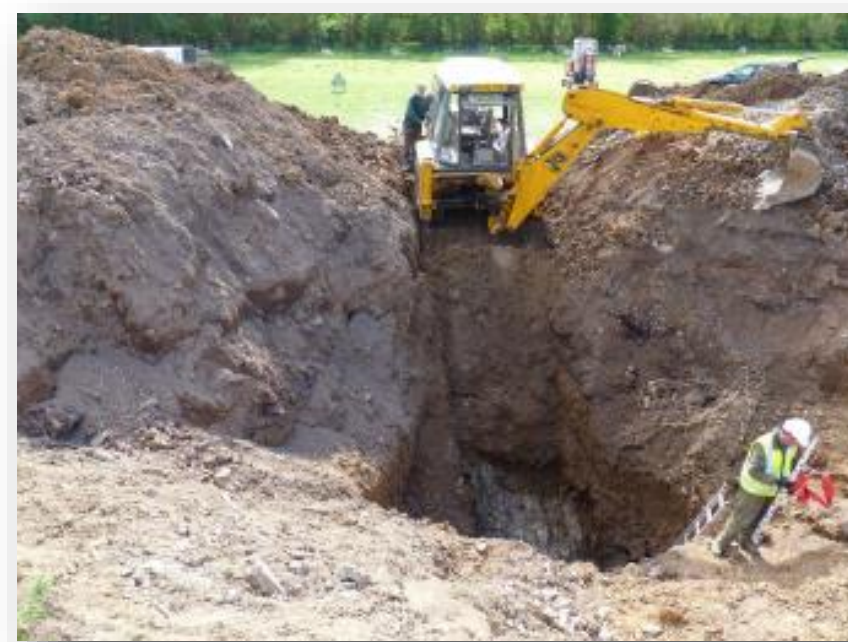
Excavation of the crater
